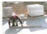
4. Drag the sand and scrap the pavers
