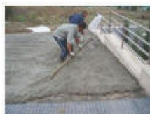
3. Concrete inclinations
