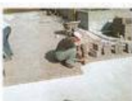
5. Installation of paving blocks
