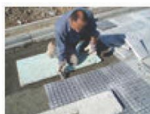
8b. Lay down the concrete tiles by using a rubber mallet
